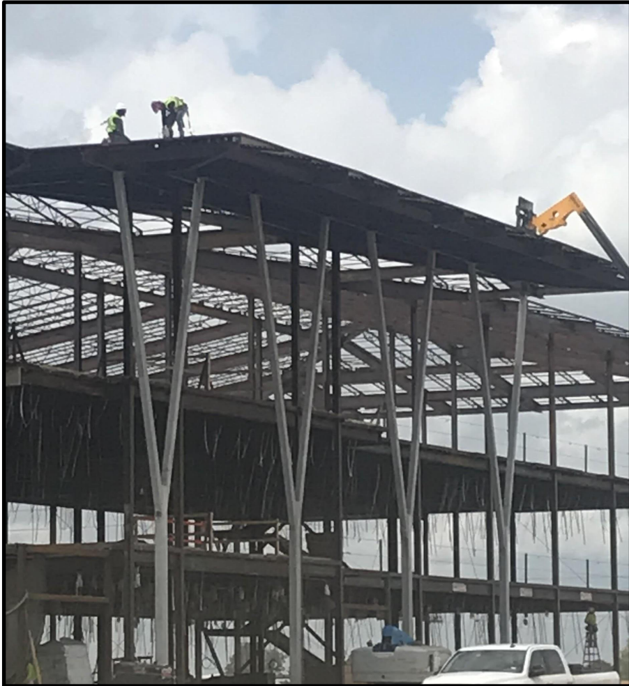
Structural Steel Erection
