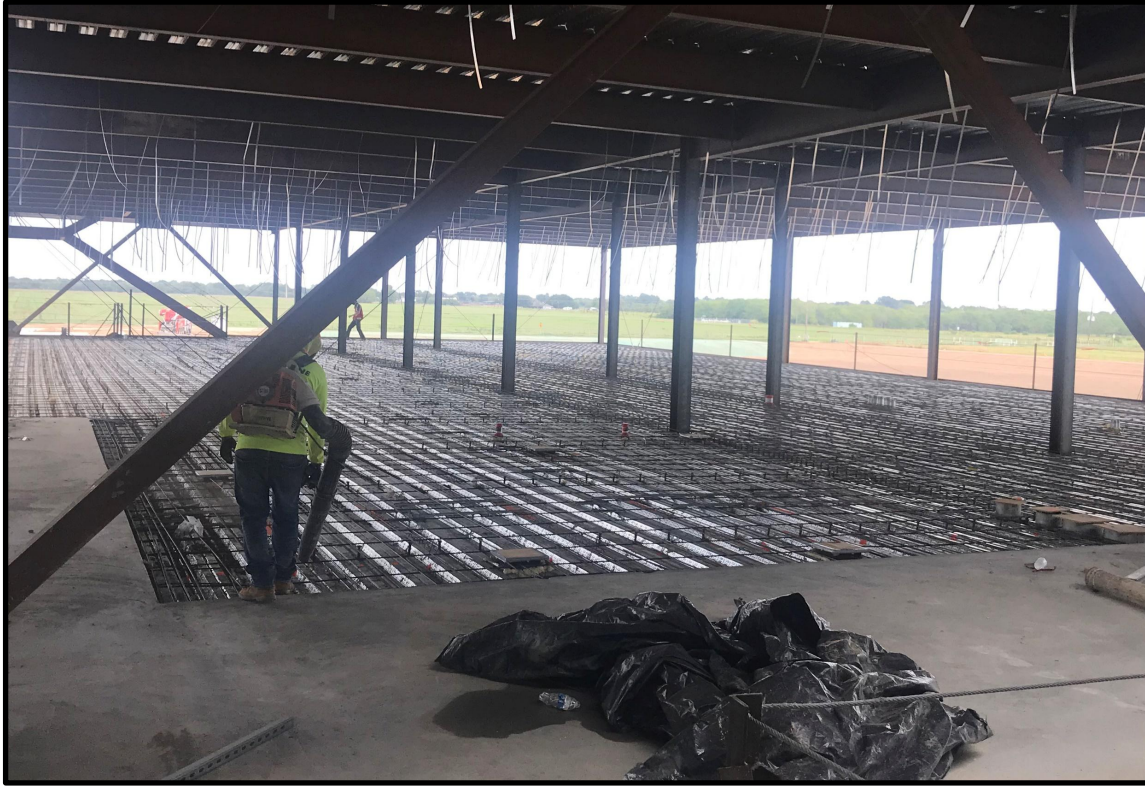
2 nd Floor Concrete on Metal Deck in Area C
