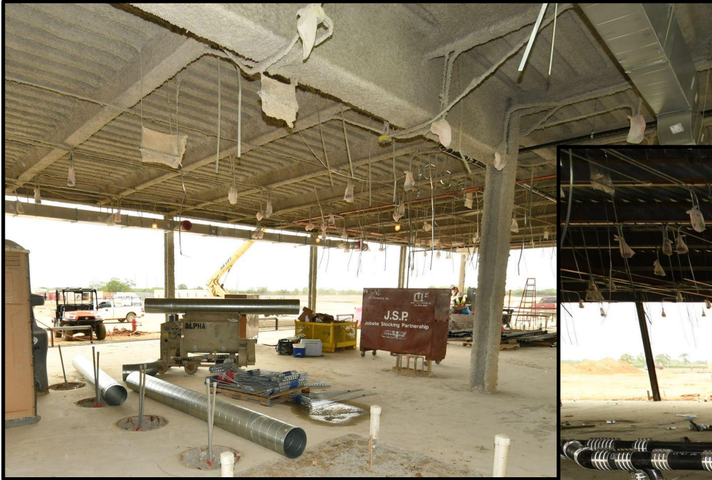
Plumbing, HVAC, and Electrical Rough-In (Fire Proofing)
